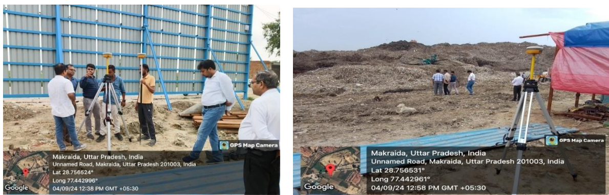
Figure 3: Contour survey at the site using Differential GPS method
