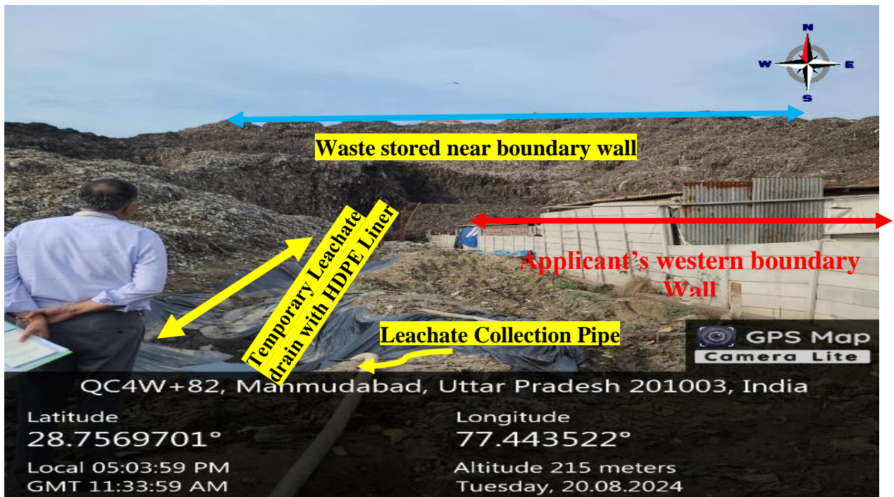
Figure 6: Temporary leachate drain along applicant’s western wall.
