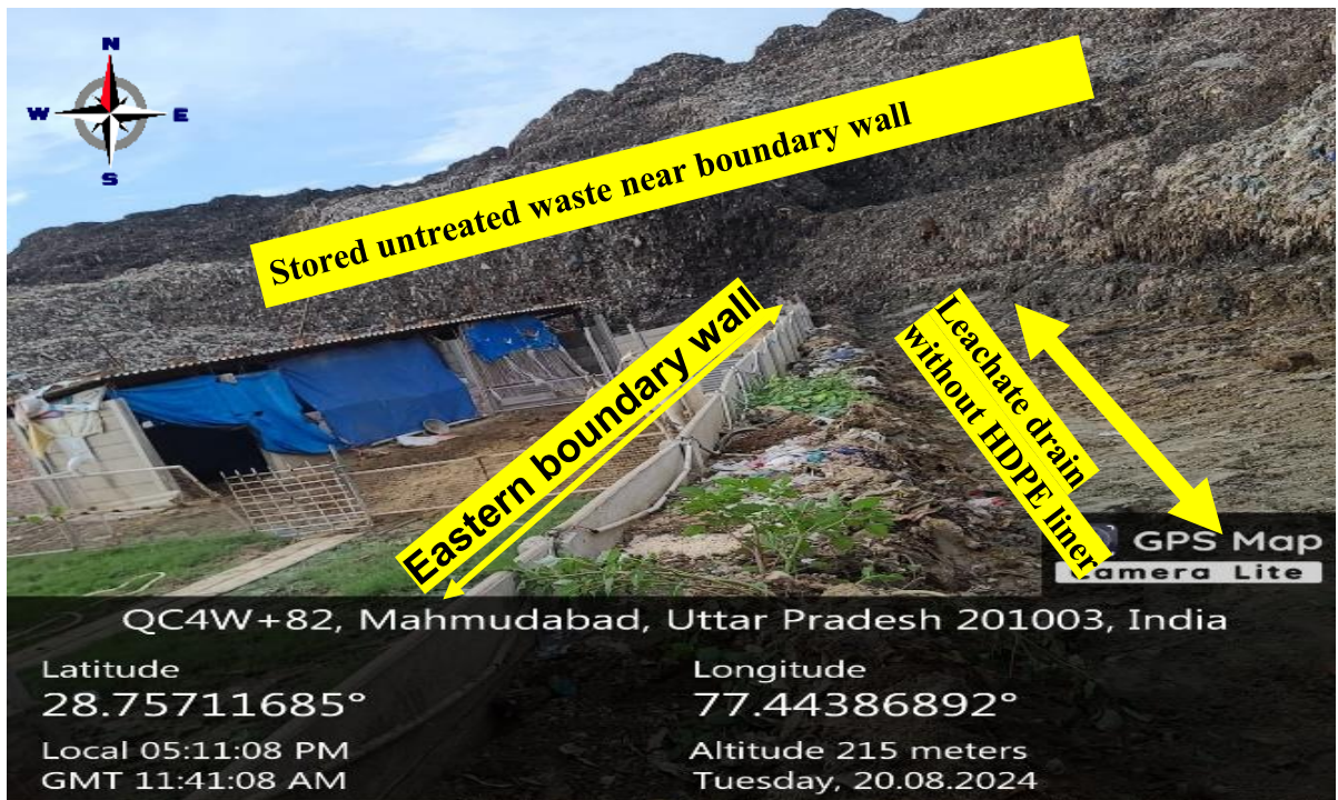
Figure 5: Waste stored is approx. 8-12 feet distance from applicant’s boundary wall
